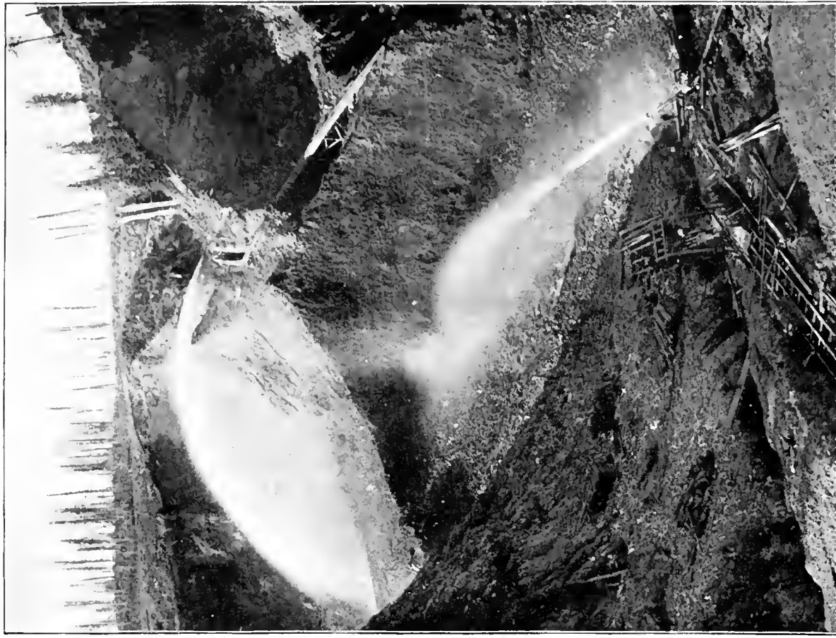
HYDRAULIC WASHING WITH MONITORS—CONSOLIDATED CARIBOO HYDRAULIC MINING CO.
